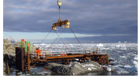
Construction work taking place
